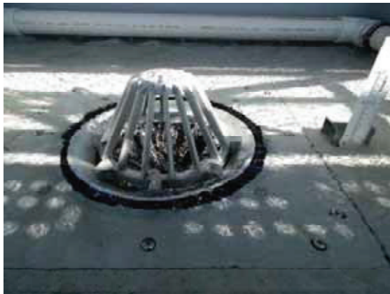
Weir Flow 18 L/s (42mm)
